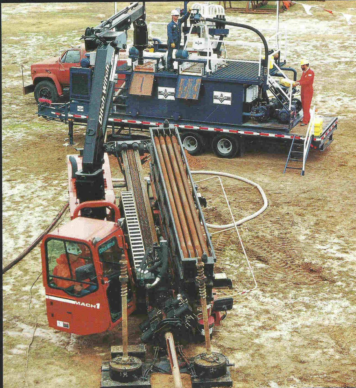
Directional Drilling with Ditch Witch, Tri-Flo and John Deere — PAGES 6-8
